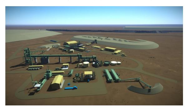
Figure 3 Plant Layout (Aerial view looking east. Processing plant in the foreground, IWL to the left (north). The ROM blending stockpiles are visible behind the plant and the Gabanintha open cut (3.2 km long) is in the background. A second waste dump is located east of the pit.
