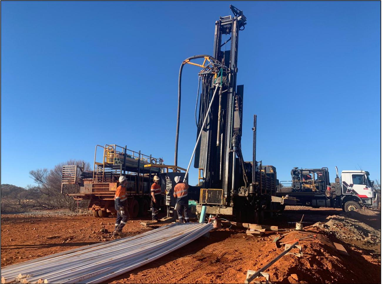
Figure 6 - Drill rig crew commence casing BBRC050 with 50mm PVC pipe
